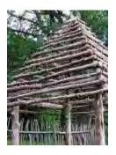
Prop up the bottom of the arbor with a block. Attach the first 40-inch-long roof slat in the middle of a top piece. Nail additional slats along one side, spacing slats 6 to 8 inches apart. Step back to check that both sides are parallel, then nail roof slats to the second gable. Add more slats on each side of the top. Cut off any excess.
