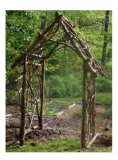
Fasten one side panel facing up to top triangle with its decorative side facing out. Set the other side up and nail it to the other end of the top. Place the second gable in place and nail from the inside of the arbor. Use two 60-inch-long sticks to form an "X" between the two gable pieces; before nailing them in place, step back to judge whether the arbor is square.
